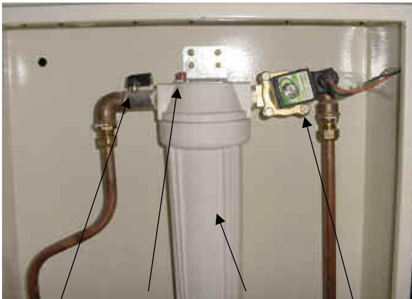
Shutoff Valve    Bleed Valve    Filter    Water Solenoid
