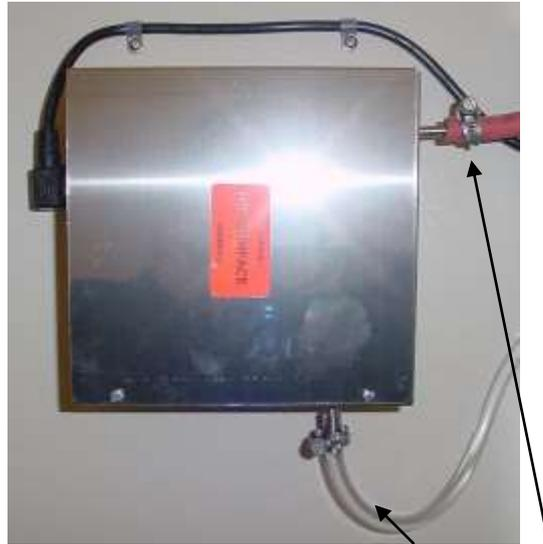
Steam Injection Module (P2003) INLET OUTLET
