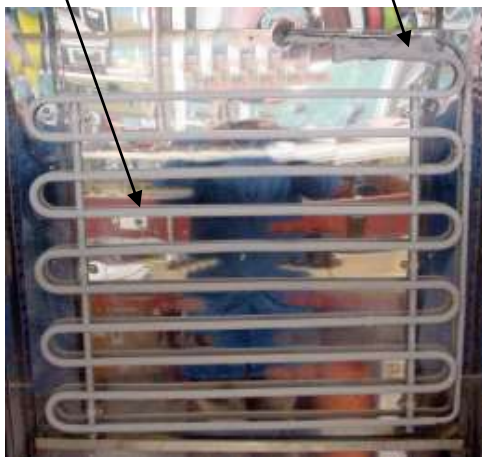
'Frosted' Evaporator & 'Frosted' Surge Pot
