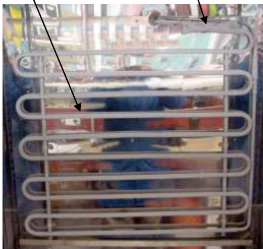
'Frosted' Evaporator & 'Frosted' Surge Pot
